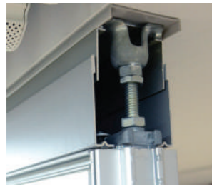
01 Ceiling & Integrated Floor Connection
